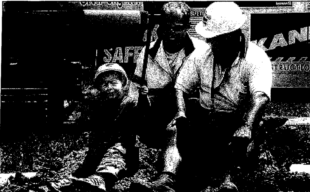
Brayden, with workers Sam Breese and Doug Putt, turns the first sod at the site of the new hospital nursery.
